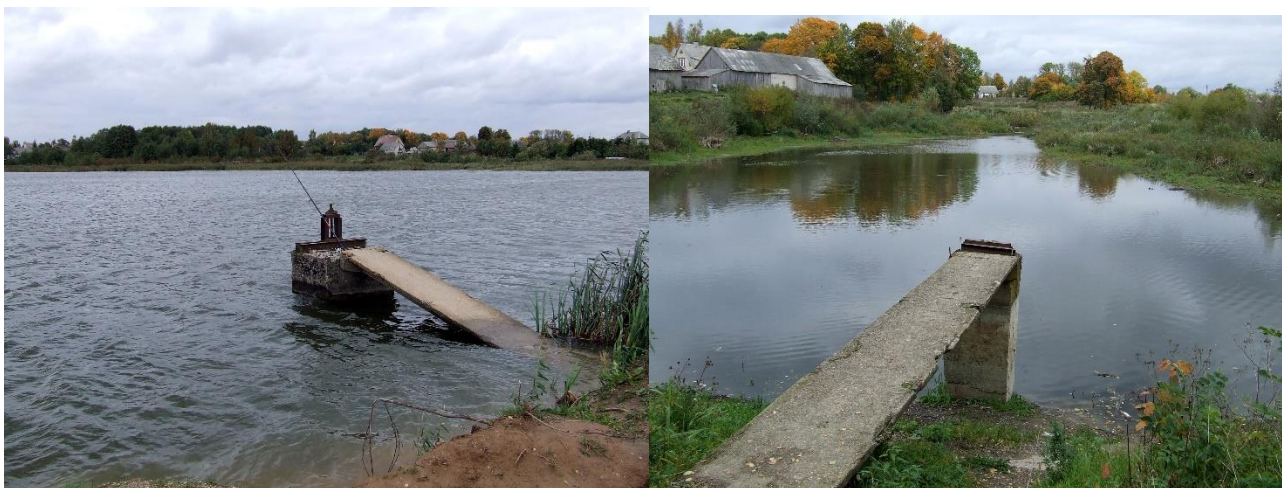
Figure 3. The shaft culverts in Gyliai I and Gyliai II abandoned hydroschemes
