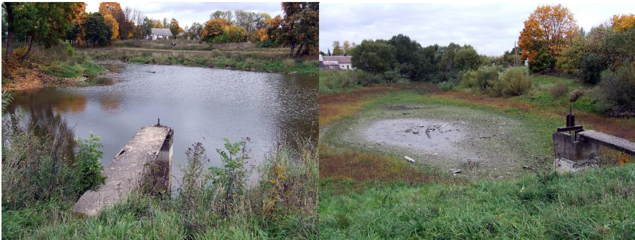
Figure 4. The shaft culverts in Gyliai III and Gyliai IV abandoned hydroschemes
