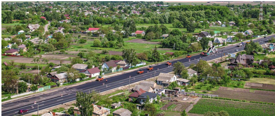
Figure 1. Construction works on the Kyiv-Chernihiv-Novyi Yarylovychi road section
